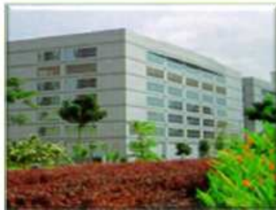
Fuel for Gas District Cooling
